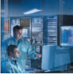
Control room of the vibration lab
